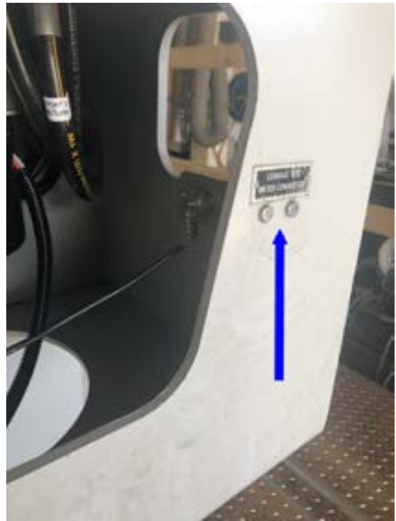
FIGURE 10 - Test port (pedestal)
